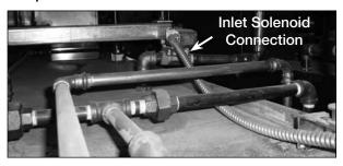
Bring the drain piping connection to the 1 in. solenoid valve in the control cabinet and connect to the threaded connection. This is a pressurized drain system and needs a properly sized drain to accommodate the pressurized drain water.
